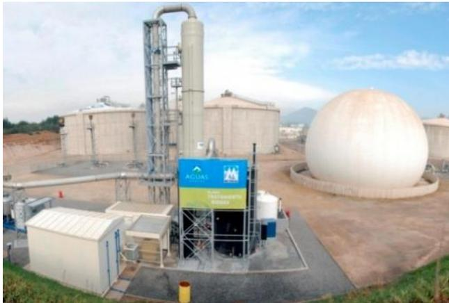
**Figure 12:** Biogas production and upgrading plant in LaFarfana, Chile (*Source: NGV Journal*)
