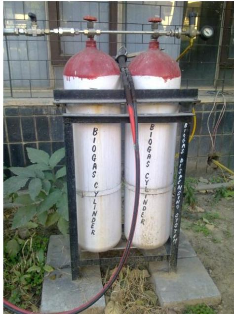
b) Two-cylinder CNG cascade
